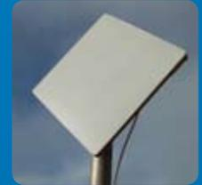
ABS - Access Base Station antenna. Co-located with the HSS antennas below roof top level
