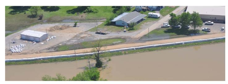
During the next ten days the river rose to the top of the wall and continued to threaten the town. The DefenCell barriers remained solid and additional barriers were installed to protect 'boils' and leaks from weak areas of the levees.
