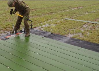
FAUN Trackway supply a kit of aluminium panels which are assembled by hand in a brickwork fashion to create a runway of any length and width to meet our customers requirements. Installation accessories and anchorage devices are also provided in the kit.
