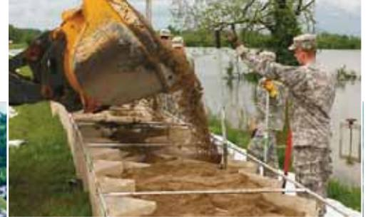
Within an hour of delivery, small teams were able to start placing, connecting and filling the systems. After just two hours, installation was being achieved at a rate of 20+ units per hour, (Equivalent to 22,196 sand bags in the initial three hours after delivery.)
