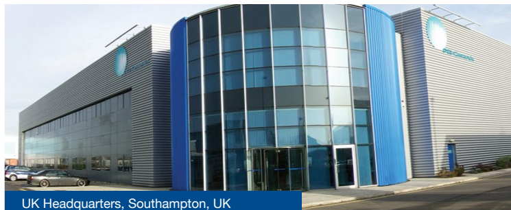
UK Headquarters, Southampton, UK
