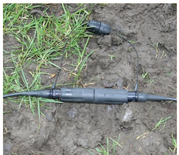
6. Connectors plugged and ready for service.
