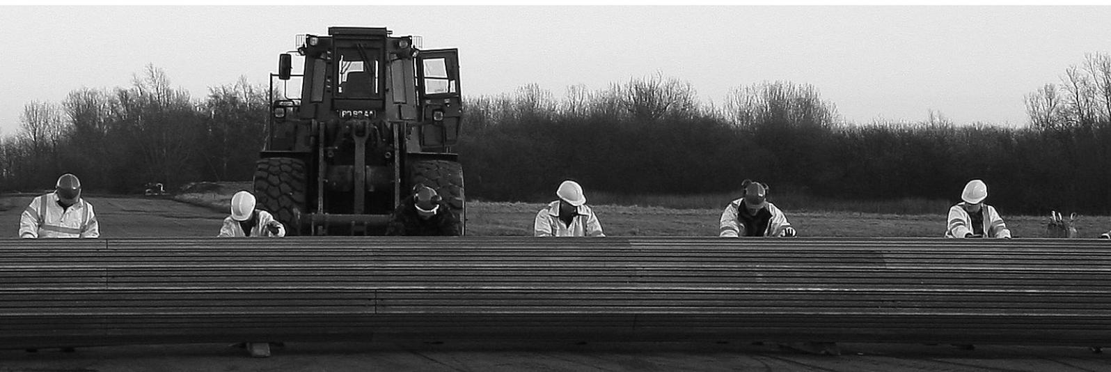
FAUN Trackway M150 panel is used to create the FAUN trackway Bomb Damage Repair Mats (BDRM) and Bomb Damage Repair Patches (BDRP) that form a vital part of the Rapid Runway Repair (RRR) process. In addition to Bomb Damage Repair Mats and Patches, FAUN Trackway also provides a complete kit for RRR to be carried out.
