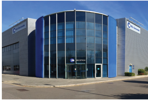
European Headquarters & Production Facility, Southampton, UK
